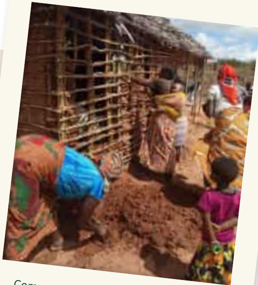
Community members make repairs to the temporary health clinic.
