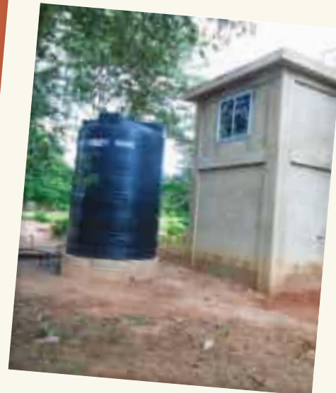
New water tank riser at Milola Secondary School.
