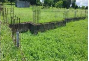
Plate No. 2.3-4: Foundation Part for the Construction of Phase II Building.
